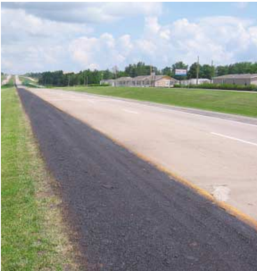
Left, the recycled shoulder on State Highway 61 in Missouri.
