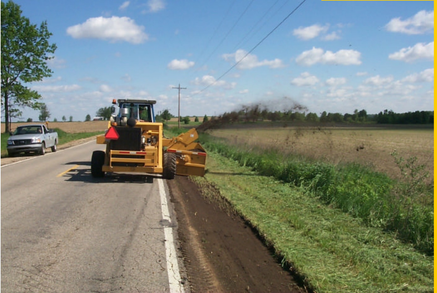
High Production Berm Removal
